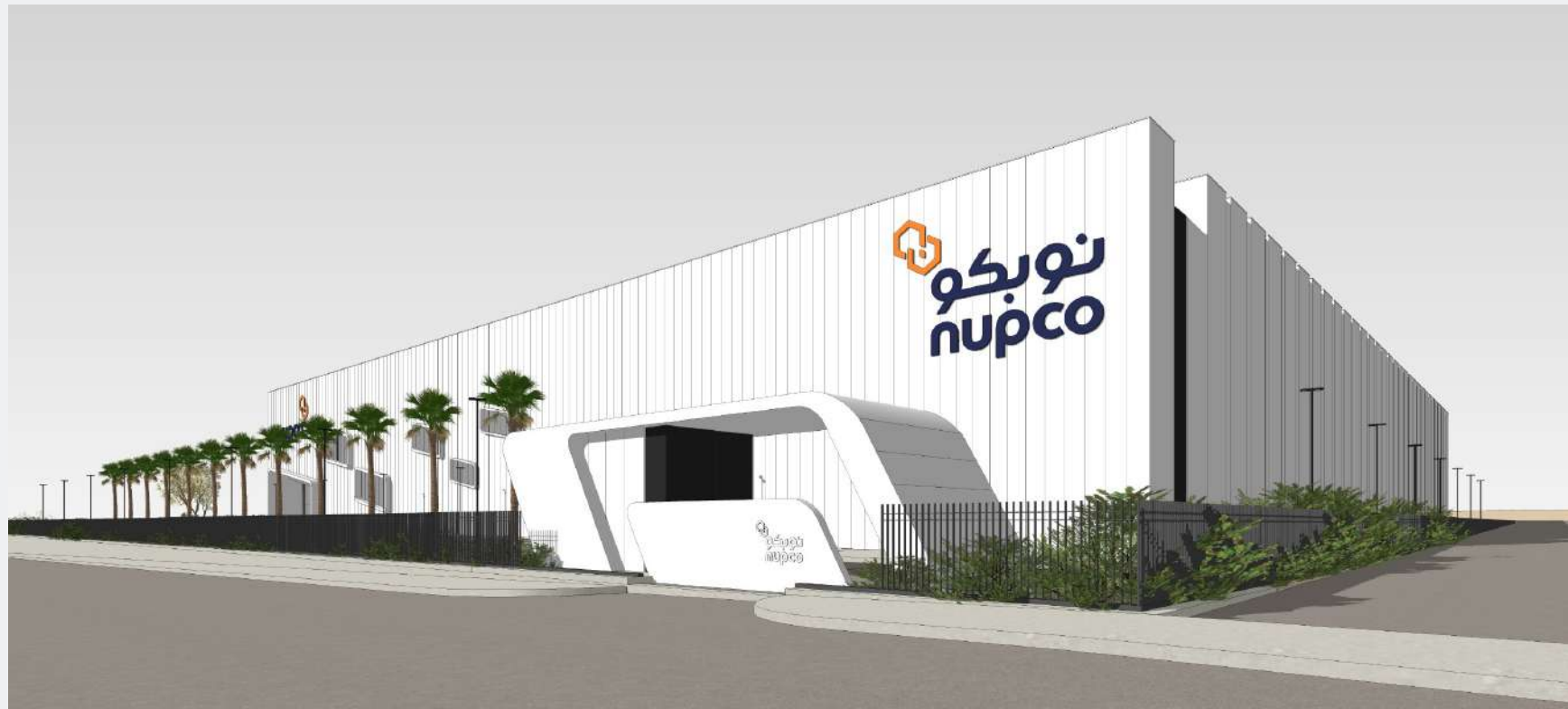
South West View – Car Entry View
